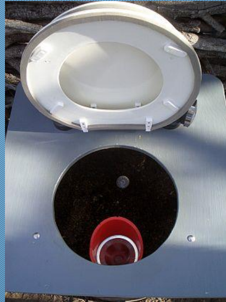
Figure 15: Urine Diversion System [2]
